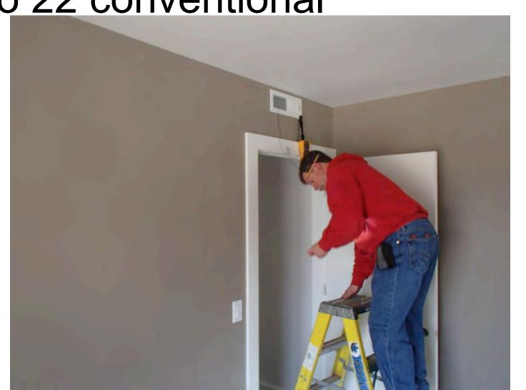
Supply air temp, ducted mini split 125 f heating /43 f cooling
