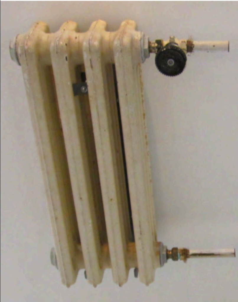
Traditional cast-iron radiator
