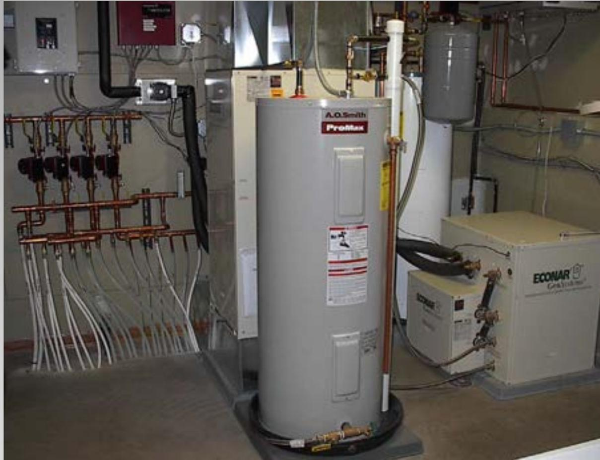
**5 T HYD GSHP w/ 3 T HYD Fan Coil combines radiant floor heating with F/A heating & cooling**
